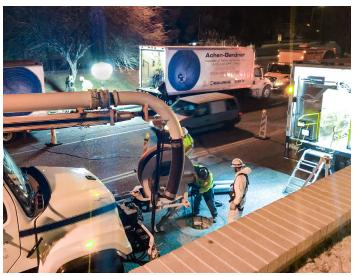
We recently completed a sewer rehabilitation in front of Banner University Medical Center in Tucson. Our ultraviolet light cured-in-place-pipe makes it possible to rehabilitate pipelines with less disruption to local stakeholders, including emergency medical personnel. This work was completed as part of our **Wastewater Conveyance JOC** project for Pima County. **Visit our website for more project information and photos.**
