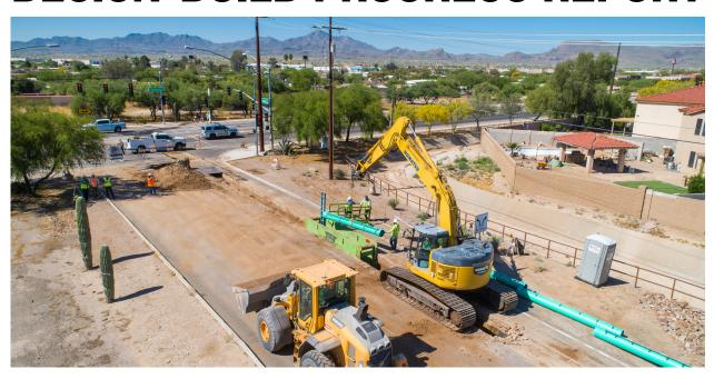
Achen-Gardner is currently constructing Segments 1 and 3 of our **Twin Peaks-Blue Bonnet Road Gravity Sewer Design-Build** project for the Pima County Regional Wastewater Reclamation Department (RWRD). These segments of the project include a total of 18,000 LF of 15" gravity sewer and 45 manholes. Segment 2 of this project, including more than 7,000 LF of 15" sewer and 12 manholes, was completed in Fall 2018. **Visit our website for more project information and photos.**
