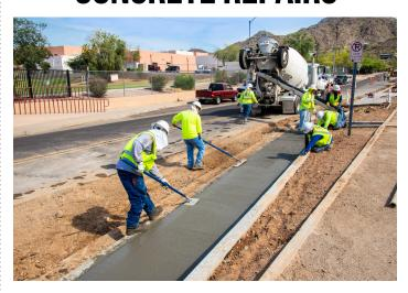
We are removing and replacing non-ADA-compliant curb ramps and repairing damaged curb, gutter, and sidewalks in front of Sunnyslope School in Phoenix. These repairs, part of our **Street Transportation Department General Construction JOC** project for the City of Phoenix, were scheduled for summer to mitigate traffic impacts around the school. **Visit our website for more project information and photos.**
