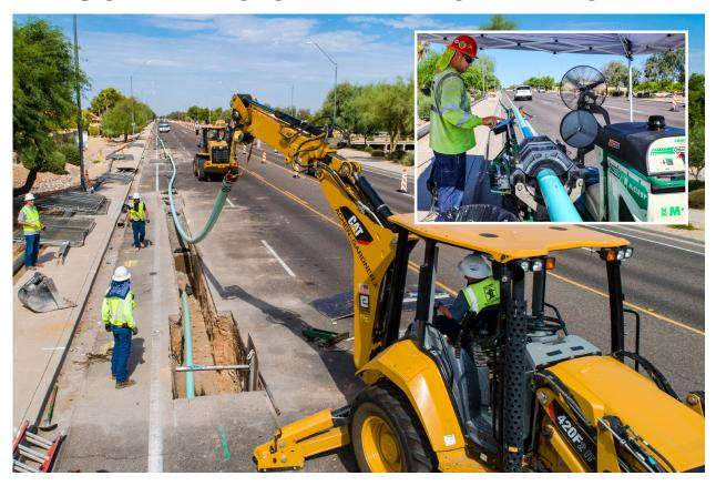
We are sliplining approximately 14,000 LF of 6" fused PVC sewer line inside an 8" ductile iron pipe from the Beardsley Road Water Relcamation Facility to 91st Avenue. We are managing 14,000 LF of bypass to support this work. This project is being completed as part of our Wet Utility Pipeline Projects JOC for the City of Peoria. **Visit our website for more information and photos.**
